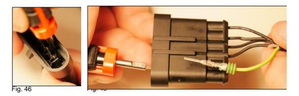
Reassemble the control panel SUPERSEAL connector and the control unit SUPERSEAL connector. Connect the control panel connector (1) to the control unit connector (2) (see Fig. 47).
